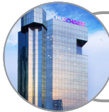
Churchgate Building, Abuja
